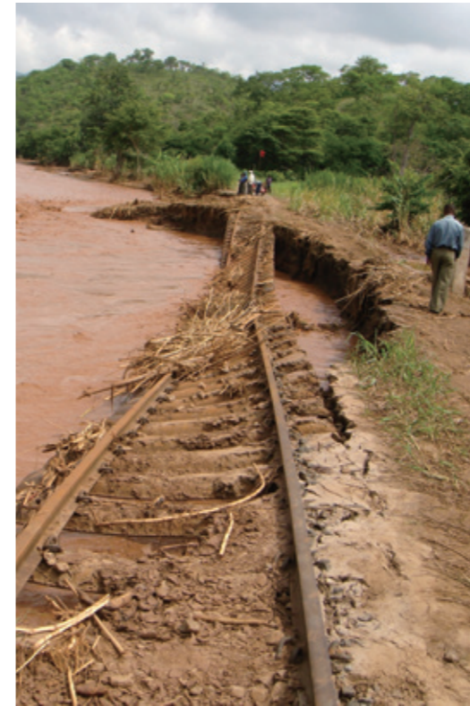
The railway tracks are planned to be relocated to the area where an erosion can hardly reach.
