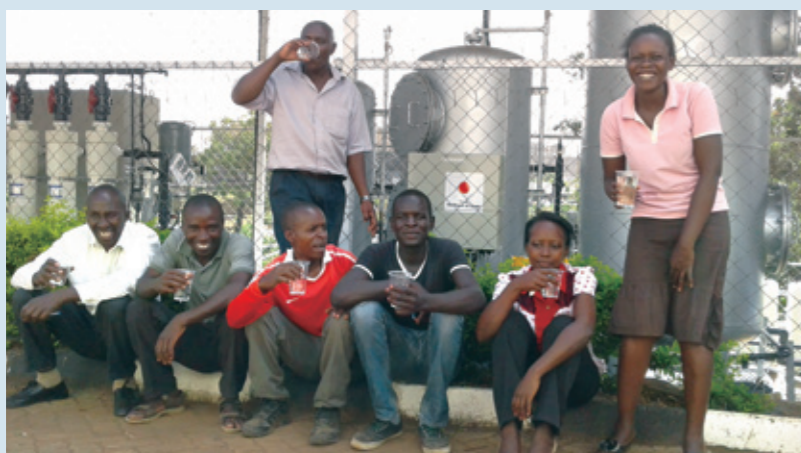
This water treatment plant provides clean water to 1,000 residents of this village.
