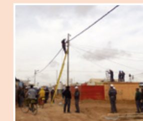
Wiring work at the Zaatari refugee camp
