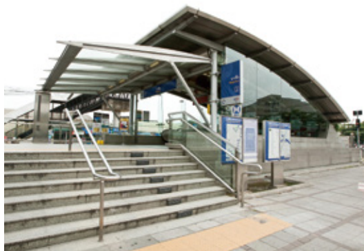
The entrance to the Bang Sue station of the MRT Blue Line. As a flood prevention measure, the station entrance is elevated from the road.
