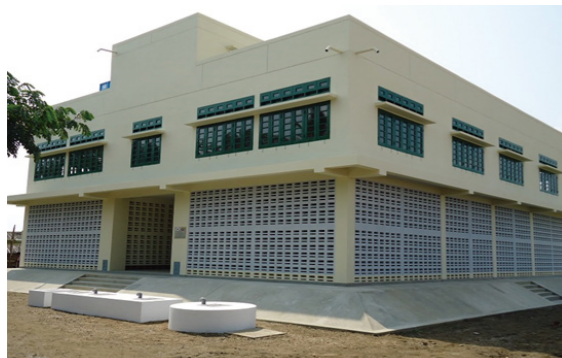
The ground floor is designed so that water can easily drain during a storm surge. The local community can evacuate to the second floor and to the rooftop.
