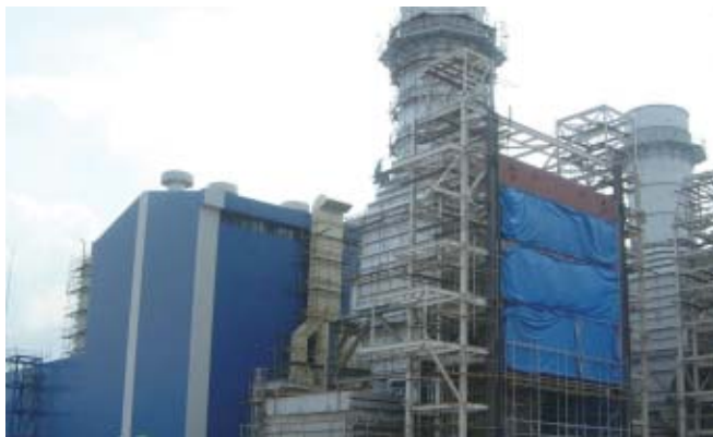
A power plant under construction in the Cilegon district, Java
