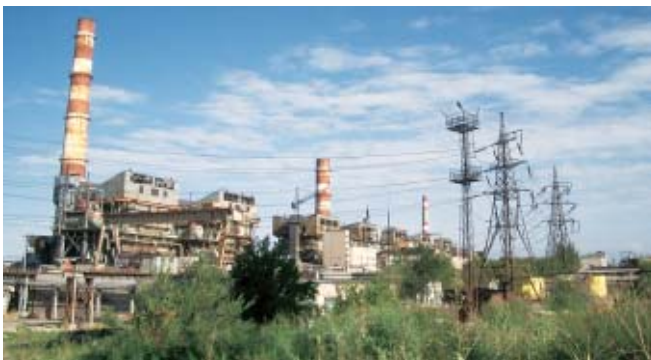
An antiquated power plant in Armenia
