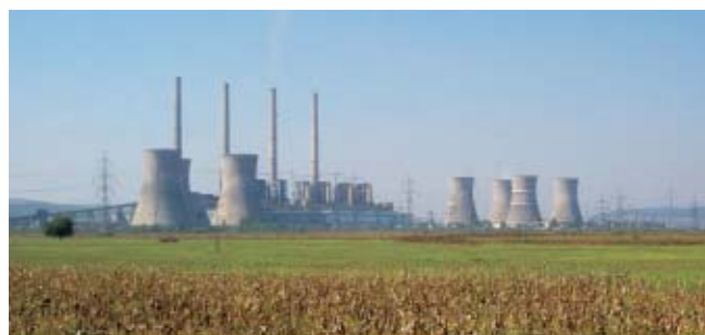
The Turceni Thermal Power Plant where the flue gas desulfurization system will be installed
