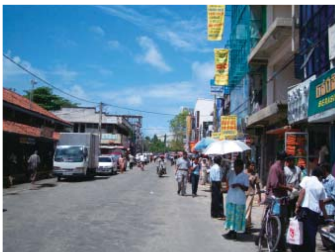
The road was improved in the first phase of the project.
