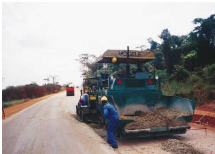
Road Rehabilitation Project
