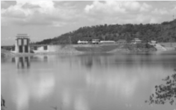
Bili-Bili Dam (Indonesia)
