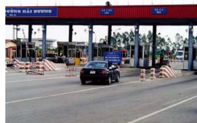
The same highway after the improvement project
