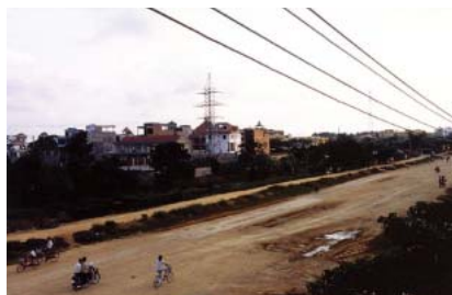
National Highway No. 5, before the improvement project
