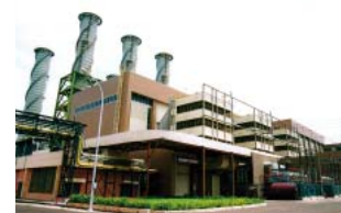
Gandhar Thermal Power Plant
