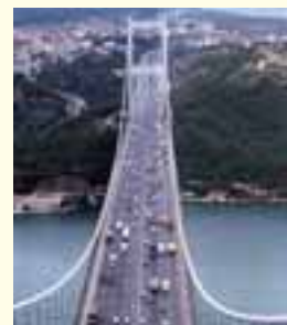
Second Bosphorus Bridge (Turkey) constructed with support from Japanese ODA loan
