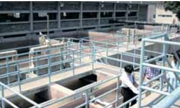
The Simly purification plant under construction
