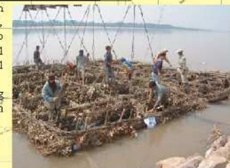
People working on the construction of Soda-matress
