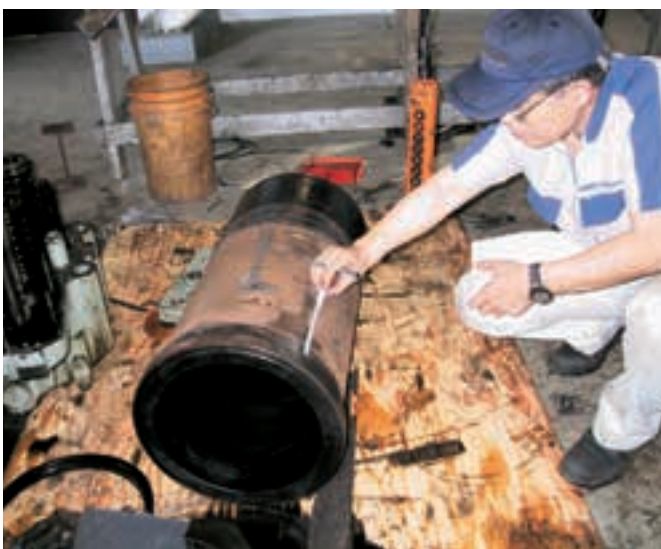
Renovation work of a power generation facility in Micronesia through follow-up cooperation
