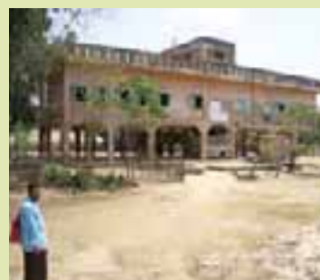
Constructed cyclone shelter
