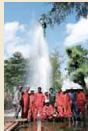
"Here comes up the water!" on-site digging training
