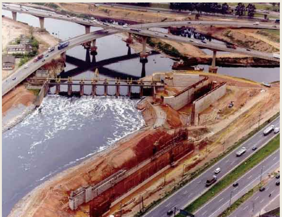
The Tiete River that runs along the main roads connecting São Paulo's Guarulhos International Airport to the city. Frequent flooding has caused extensive damage.
