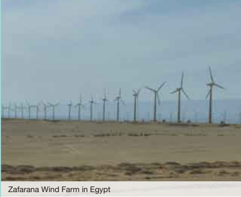
Zafarana Wind Farm in Egypt
