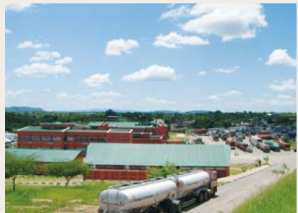
A new freight terminal completed at the Chirundu OSBP. The large reduction in border-crossing times is expected to yield various spillover effects including but not limited to improved commercial value of agricultural products, as a result of reduced transport cost.
