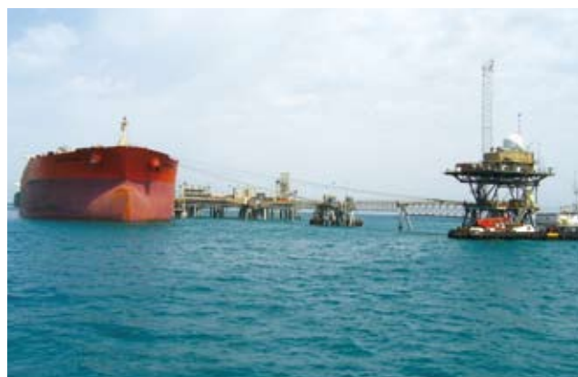
Offshore crude export terminal from which about 80% of crude oil exports are shipped from Iraq; export capacity will be doubled as a result of aid provided through an ODA Loan project.
