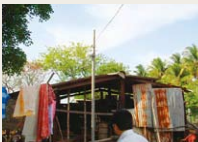
Installing an early warning system. The early warning siren for floods prevented loss of human life in this village.
