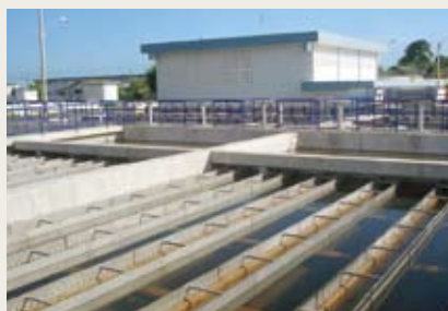
Water treatment plant after improvements
