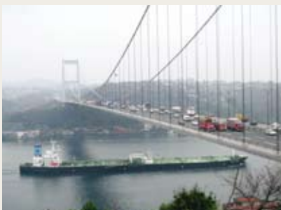
Second Bosphorus Bridge in Turkey
