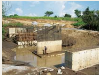
Construction site of bridge linking Otwee and Anaka
