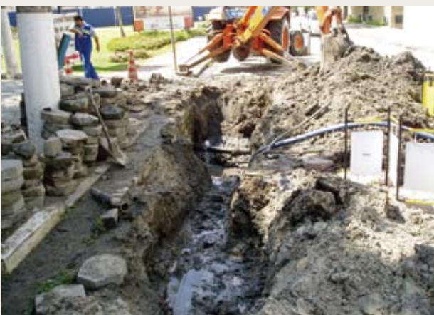
Water leak and repair
