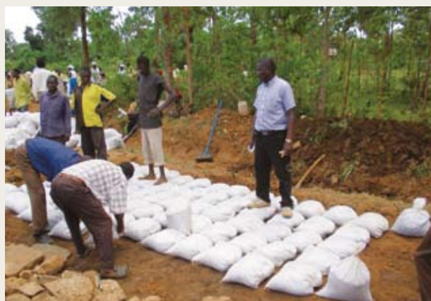
A farmers’ group restores a road in the village using sandbags. The act of cooperation helped to unify the group.
