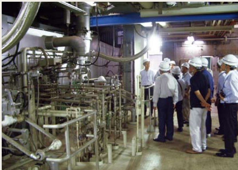
Training in Japan includes lectures and a tour of a thermal power station given by company employees.
