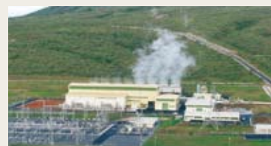
Existing Olkaria II Geothermal Power Station in operation
