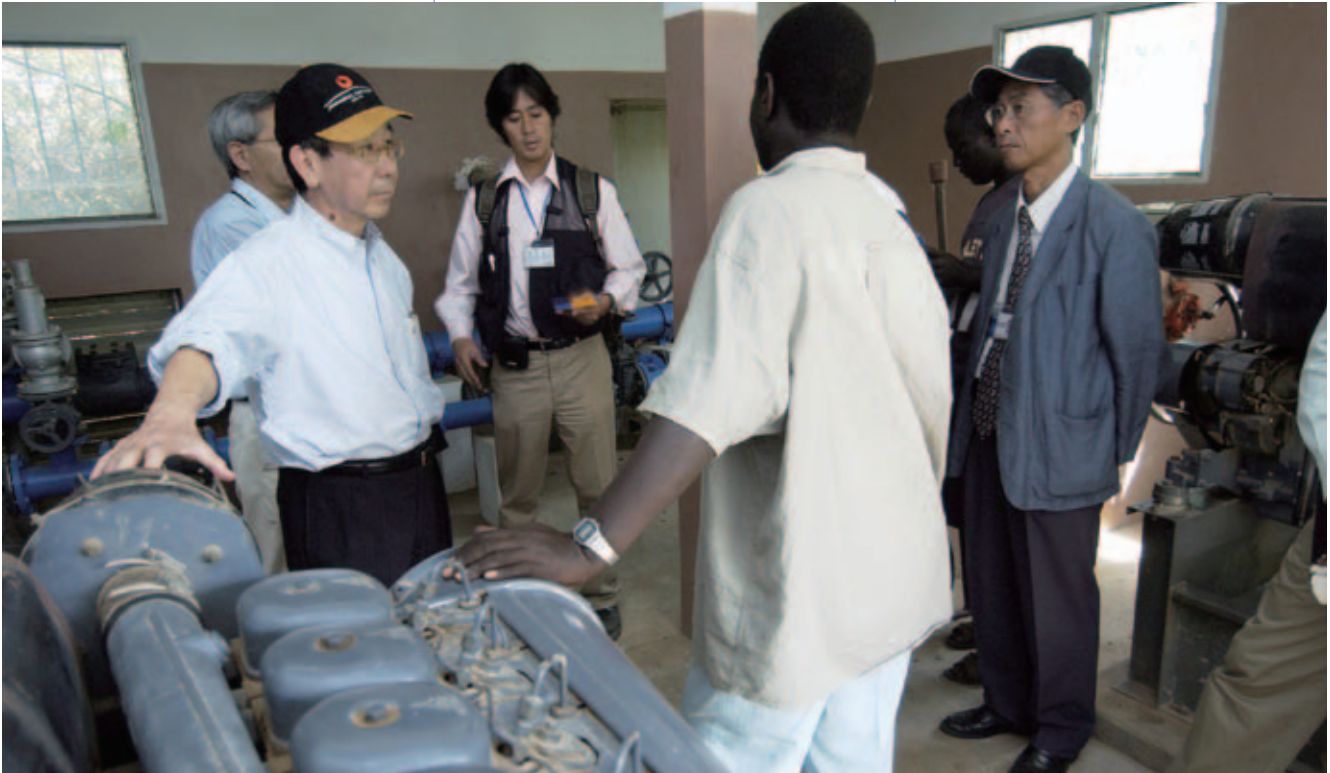
A study team checking on the maintenance conditions of a water tower/pump facility that was built with Japanese assistance. The facility is managed by a water management union that is organized by residents [Photo by Kenshiro Imamura]
