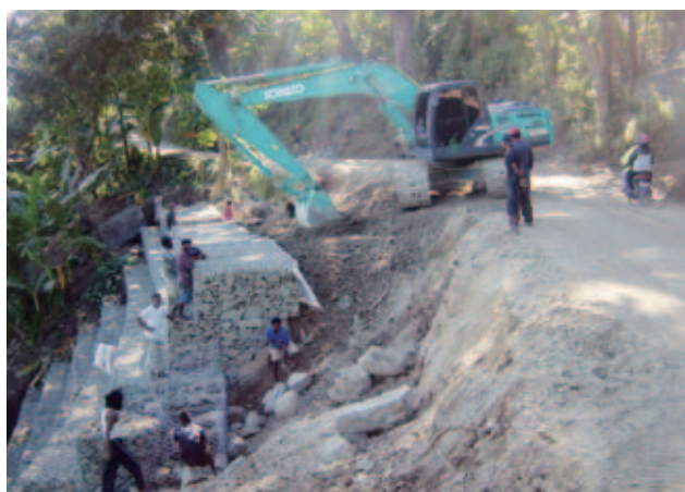
Roads are frequently blocked due to road surface damages from heavy rainfall during the rainy season (photo is of the Government’s restoration work). JICA supports capacity building in road maintenance work (Timor-Leste).
