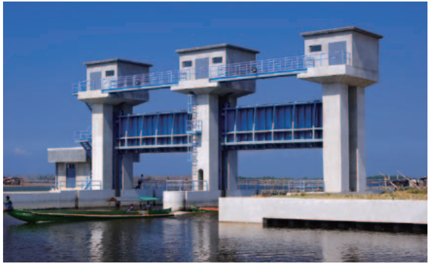
Lying on lowland terrain and susceptible to frequent flood damages, the Kamanava area in the Metro Manila, the Philippines, was installed with floodgate (photo) and drains, etc. by ODA Loans.
