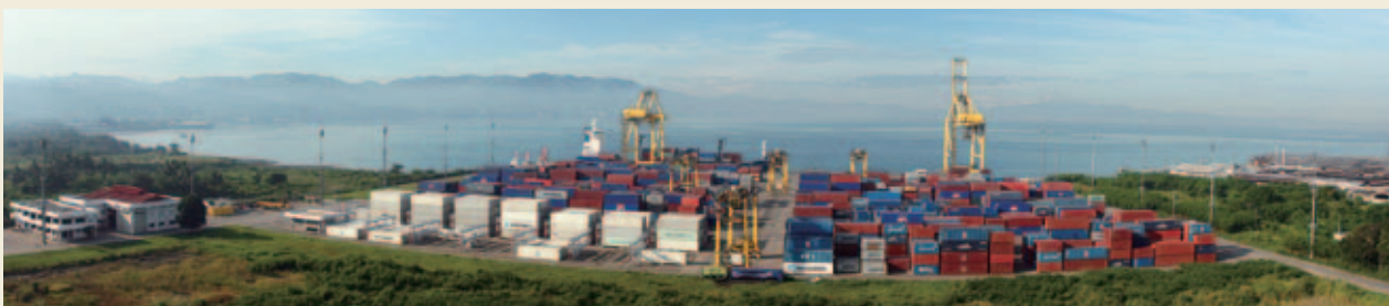
Mindanao Container Terminal
