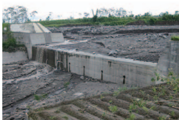
The sabo dam constructed with JICA cooperation preventing debris flow after the eruption of Mt. Merapi (Indonesia)
