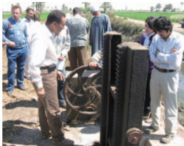
Conduit repair work at a pilot site being carried out together with an irrigation association (Water Management Improvement Plan Phase II in Egypt).
