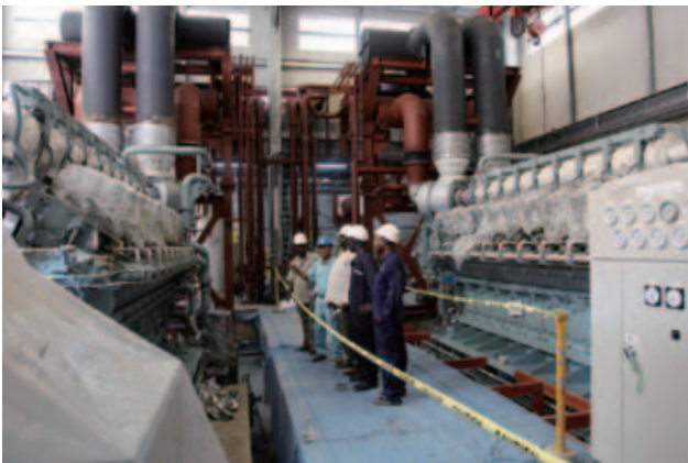
The Project for Urgent Improvement of the Electric Power Supply System in Freetown in Sierra Leone
