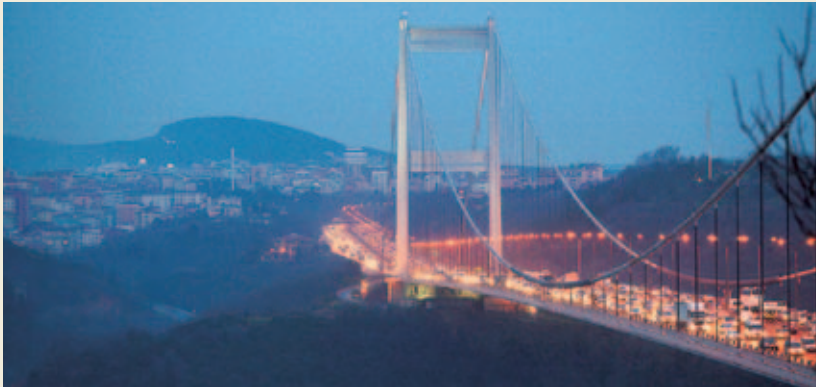
Large-scale bridges in Istanbul for which seismic reinforcement work has been completed.
