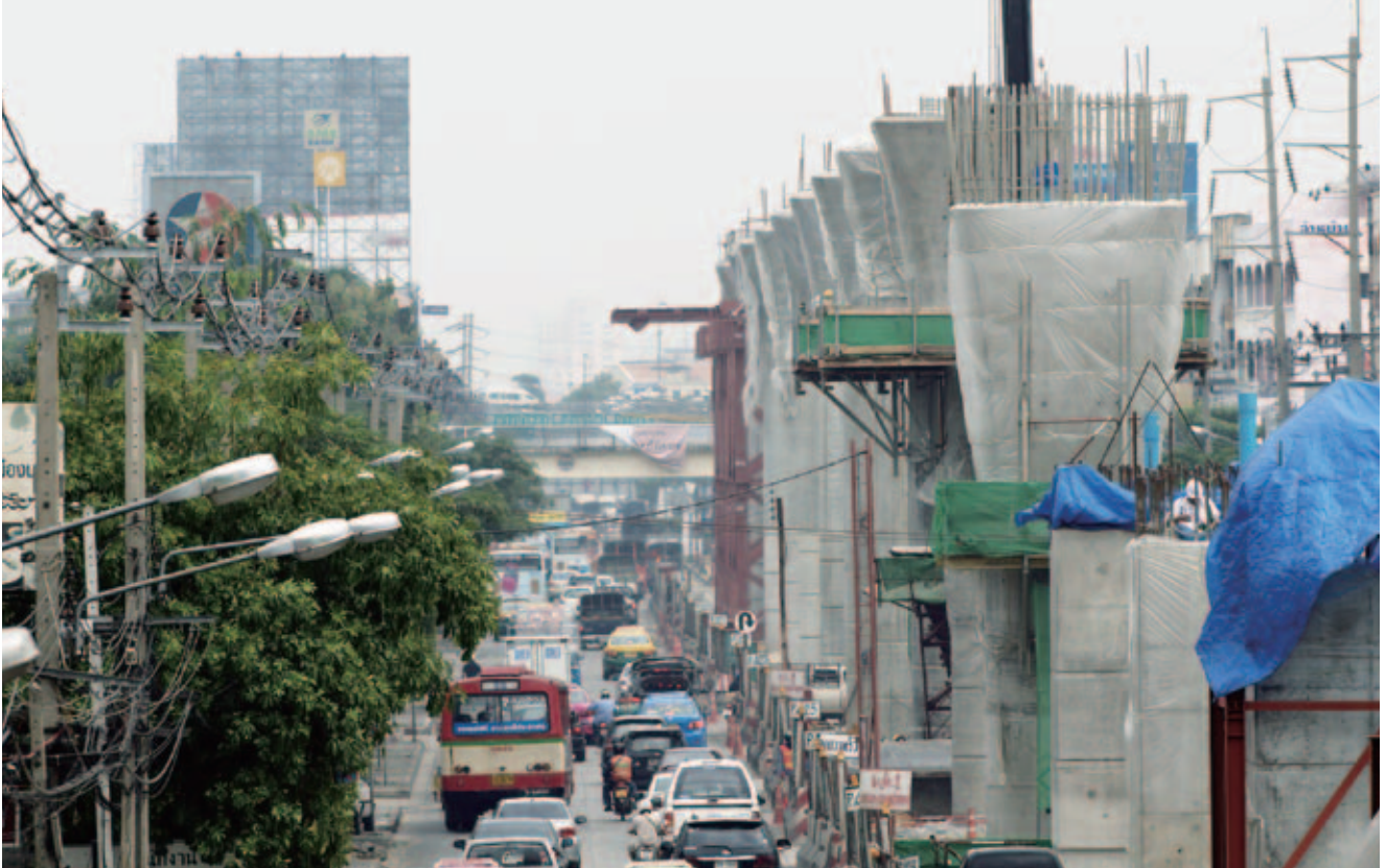
In the capital city of Bangkok, Thailand, the purple line of the mass transit system, connecting Bangkok and the neighboring Nonthaburi Province, is being constructed with the provision of ODA Loans.
