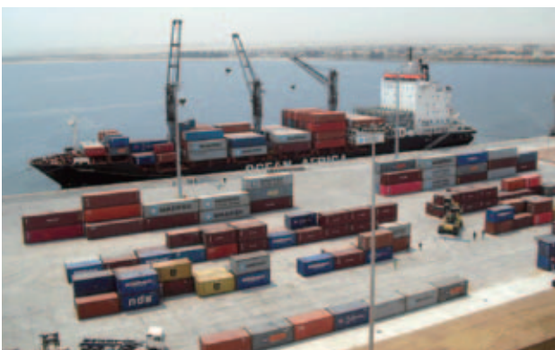
Namibe Port in Angola which was repaired with Grant Aid
