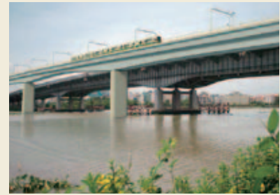
An image of an elevated bridge which crosses Saigon River, heading from central Ho Chi Minh City toward the suburbs
