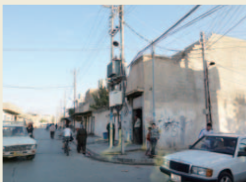
Equipment for distribution of electricity, provided via an ODA Loan (Erbil, northern part of Iraq (Kurdistan region))
