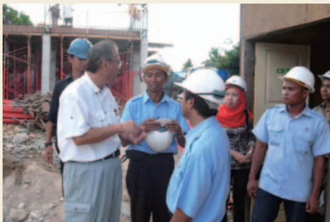
A Japanese expert providing guidance on earthquake-resistant design to local workers at the construction site.
