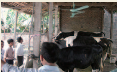
Cooling fans and anti-moisture devices were installed on the ceilings of cattle barns without walls as a heat management measure.
