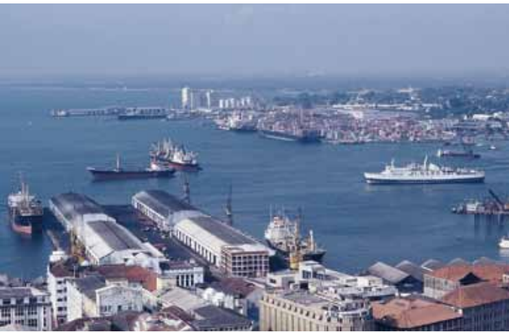
Port of Colombo North Pier Development Project (1) in Sri Lanka
