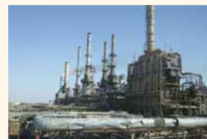
The Basrah Oil Refinery
