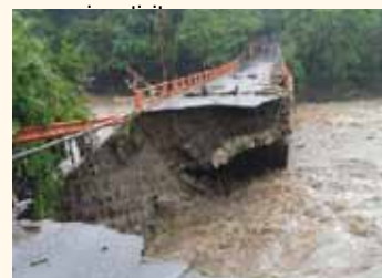
Runoff from heavy rain washed away part of the downstream side of this bridge, which was closed off by nearby residents.
