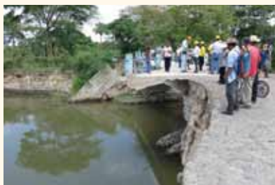
The La Zorra Bridge in La Paz Province in southern El Salvador was damaged by rain from a tropical depression in October 2011.
