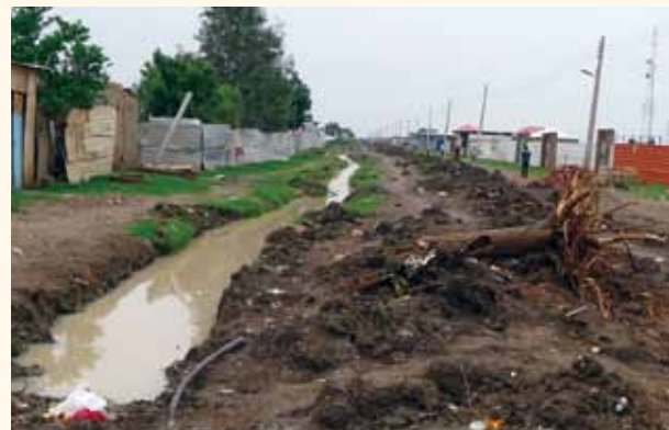
Malakal Town has almost no paved streets and the city’s so-called “black cotton soil” makes streets impassable even to four-wheel-drive vehicles and donkeys during the monsoon. This turns the city into a virtual land-locked island.
