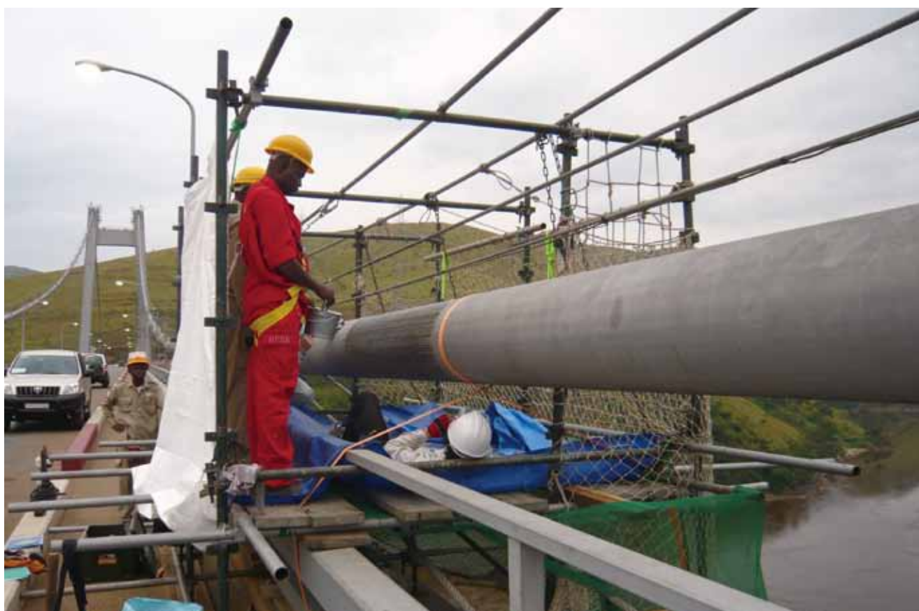
Engineers examine cables of the Matadi Bridge in the Republic of the Congo, which was constructed about 30 years ago with an ODA Loan. The bridge is still properly maintained after all these years.
