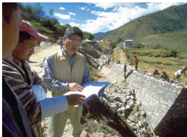
A Senior Volunteer for road maintenance and management was sent to Bhutan, where expanding the infrastructure is the highest priority. A rush highway construction project is under construction that will create a link to Thimphu, the capital of Bhutan. (Photo by Kazuyoshi Nomachi)
