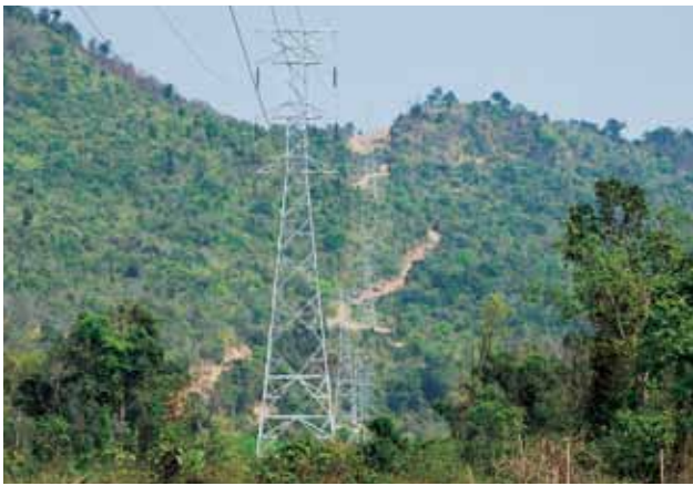
This transmission line of about 40km goes from the Paksan substation and over the Pakkading Pass.
