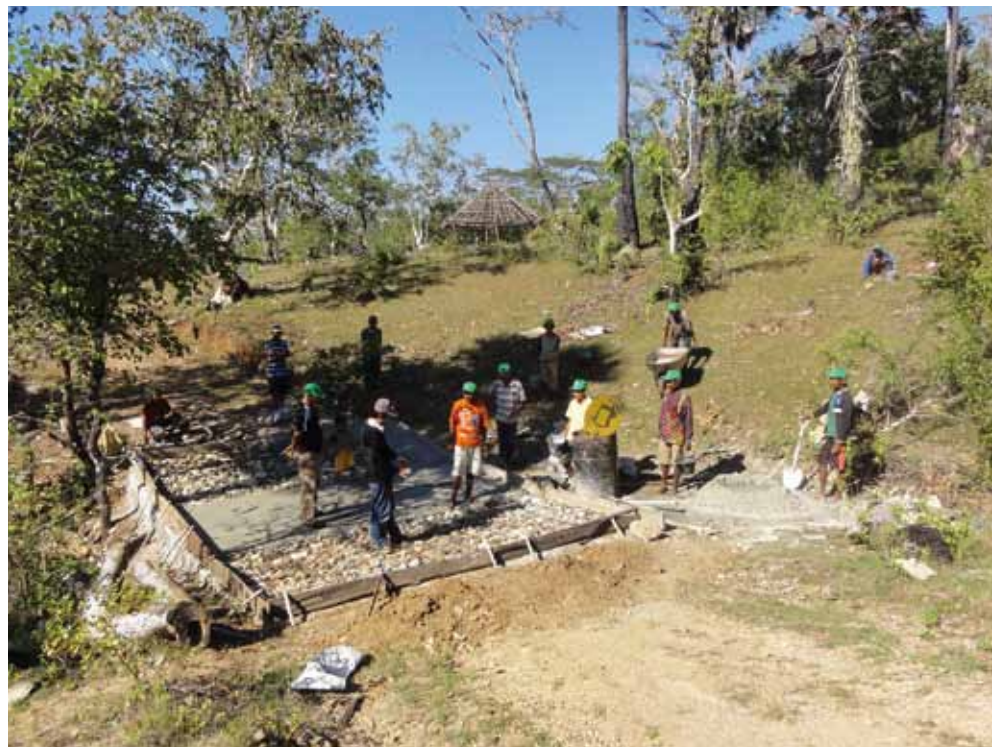
Residents build a community road (Timor-Leste)
