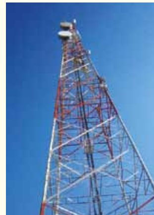
A Tower for Telecommunication in Yangon
