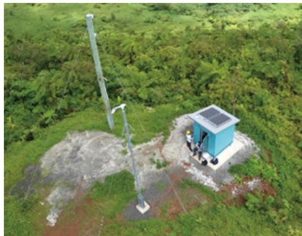
Establishment of a weather observation facility in Samoa under Grant Aid
