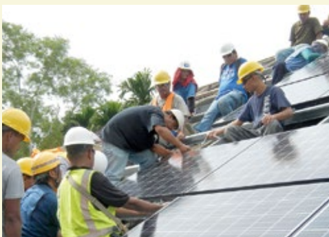
Installation of solar panels in Micronesia
