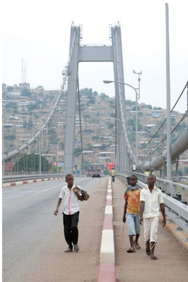
The only bridge over the Congo River, built by ODA Loan in 1983. JICA is currently providing support to enhance the maintenance capability of the bridge. (Photo by Shinichi Kuno)
