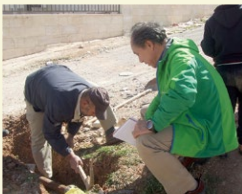
JICA expert checking the condition of a water distribution pipe in the situation analysis on water and sewerage services in host communities.
