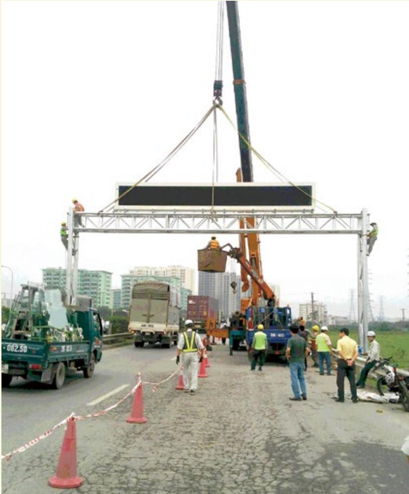
Installing a traffic control system provided under Grant Aid on a highway in Hanoi, Viet Nam.
