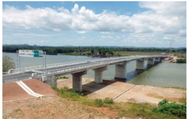
The Santa Fe Bridge, spanning the border between Nicaragua and Costa Rica, is expected to play a role in accelerating international logistics. (Project for Construction of the Santa Fe Bridge in Nicaragua)
